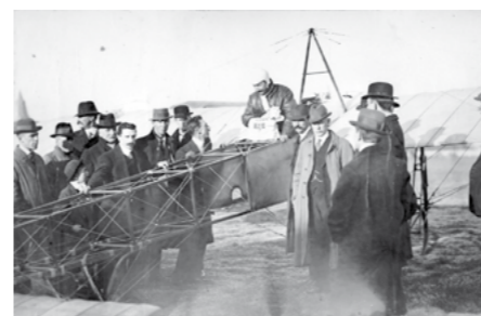
The first airmail service within Australia occurred in this bi-plane in 1914.
