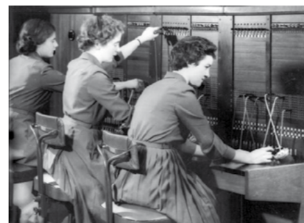
A busy telephone exchange in Melbourne in the 1940s.
